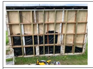
The back of the hut with cladding removed. Two pieces had already fallen off. Oddly, the main lengths of structural timber were horizontal, with shorter lengths in between making up the vertical support. (Alex and I have walked on the roof more than once when fitting the wind turbine and racing light systems.)
